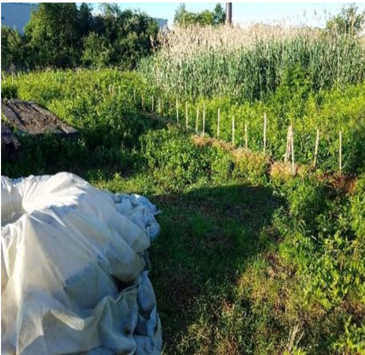
Fig 3: Straw bales installed between Str. 193 and wetland NW37. Viewing southwest. (7-01-19).
