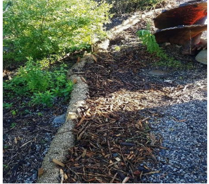
Fig 2: Combined berm installed in laydown area off of Gosling Rd cont. Viewing north. (7-01-19).
