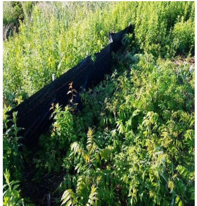
Fig 6: Silt fence installed between Str. 137 and wetland NW37 cont. Viewing east. (7-01-19).
