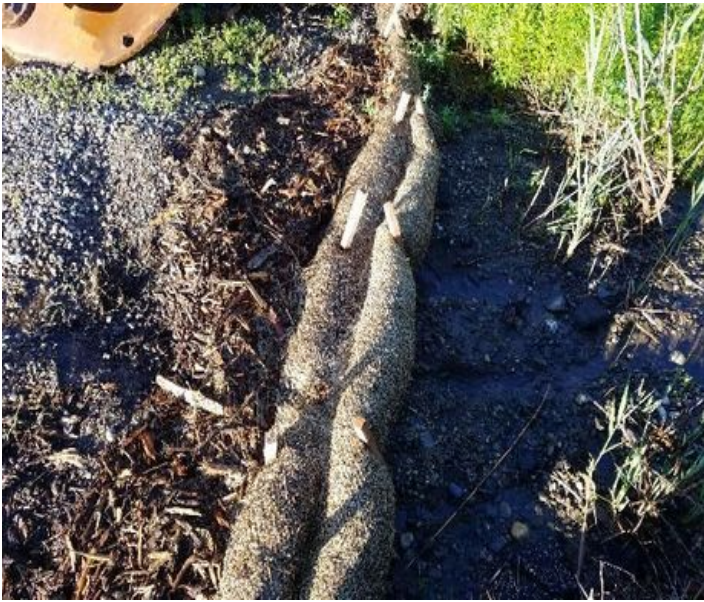
Fig 1: Combined berm installed in laydown area off of Gosling Rd. Viewing south. (7-01-19).
