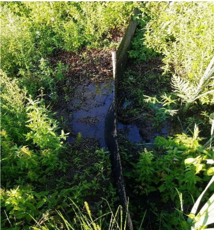
Fig 7: Silt fence installed between Str. 137 and wetland NW37 cont. Viewing east. (7-01-19).
