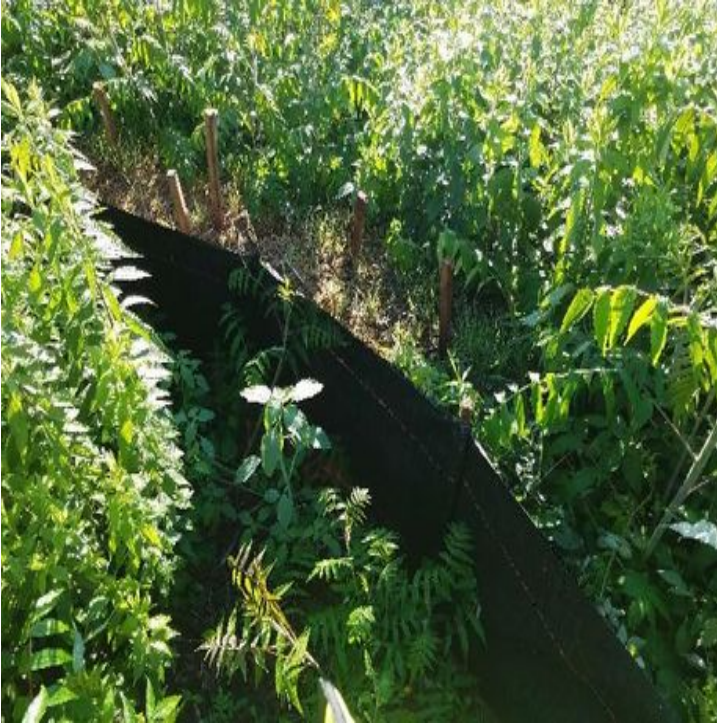
Fig 5: Silt fence installed between Str. 137 and wetland NW37. Viewing west. (7-01-19).
